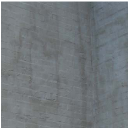
Examples of mottled, blotchy and streaky effect produced by cementitious products
